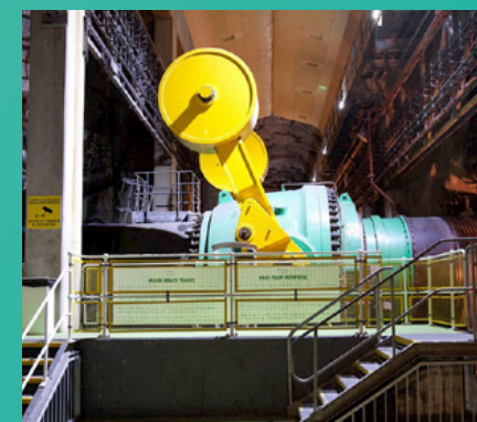
The main inlet valve at Dinorwig, Wales
