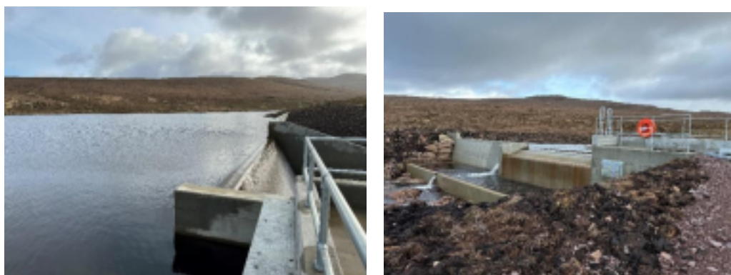
Figure 2 – intake to penstock from Reservoir
