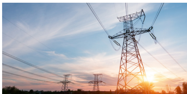
Transmission constraints pose a barrier to net zero, we need to accelerate innovation to enable us to 'sweat' our current assets.
