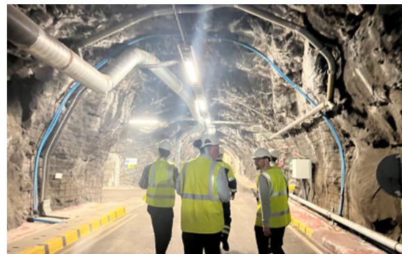
The subterranean access tunnel at Cruachan
