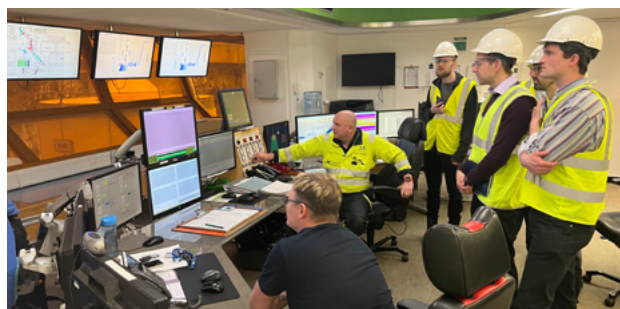
The Control room at the Cruachan facility.
