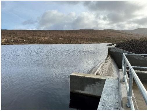
Figure 2 – intake to penstock from Reservoir
