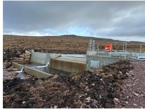
Figure 2 – intake to penstock from Reservoir
